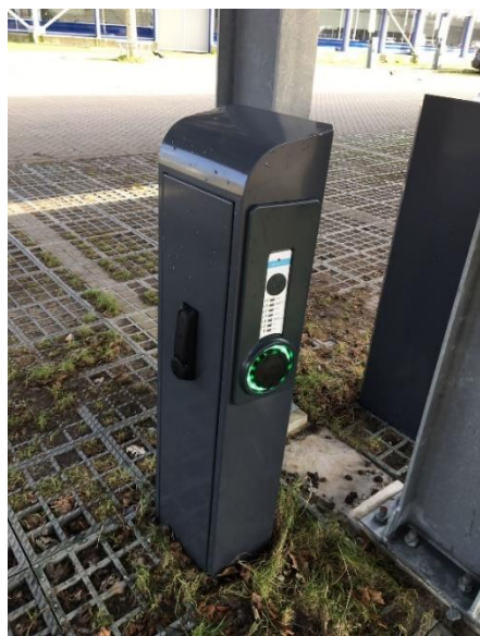
Figure 16: Charging stations for cars and bicycles
