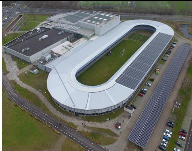
Figure 11 :Top-down view of ‘De Meent’ sports centre ( https://sun-projects.nl/ )
