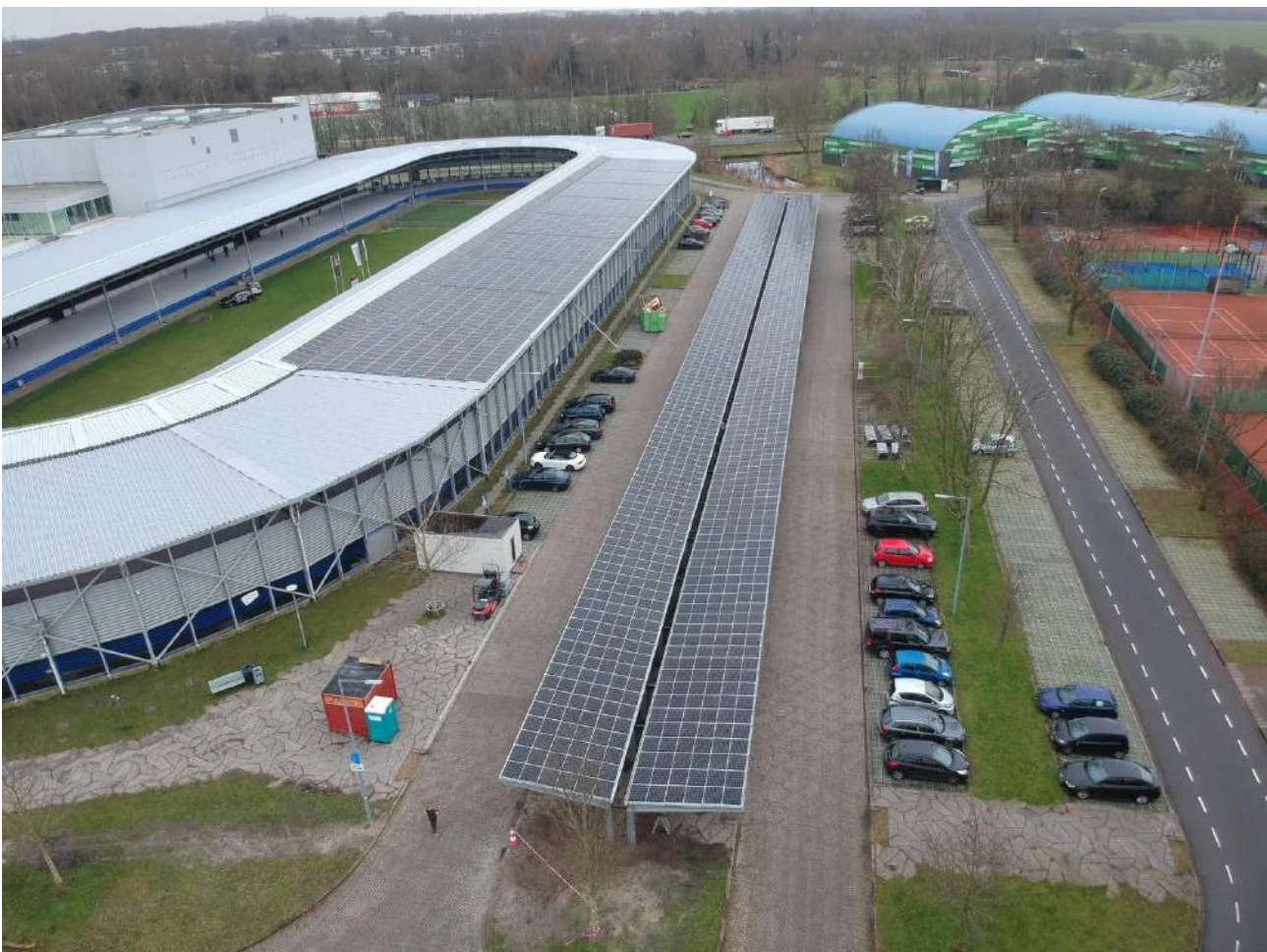
Figure 4: PEB 1.1 - De Meent with installed PV panels above the car port
