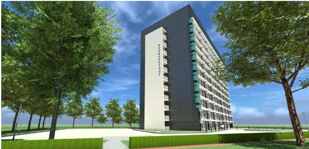
Figure 5: Woonwaard Highrise van der Veldelaan with visualization of the solar construction
