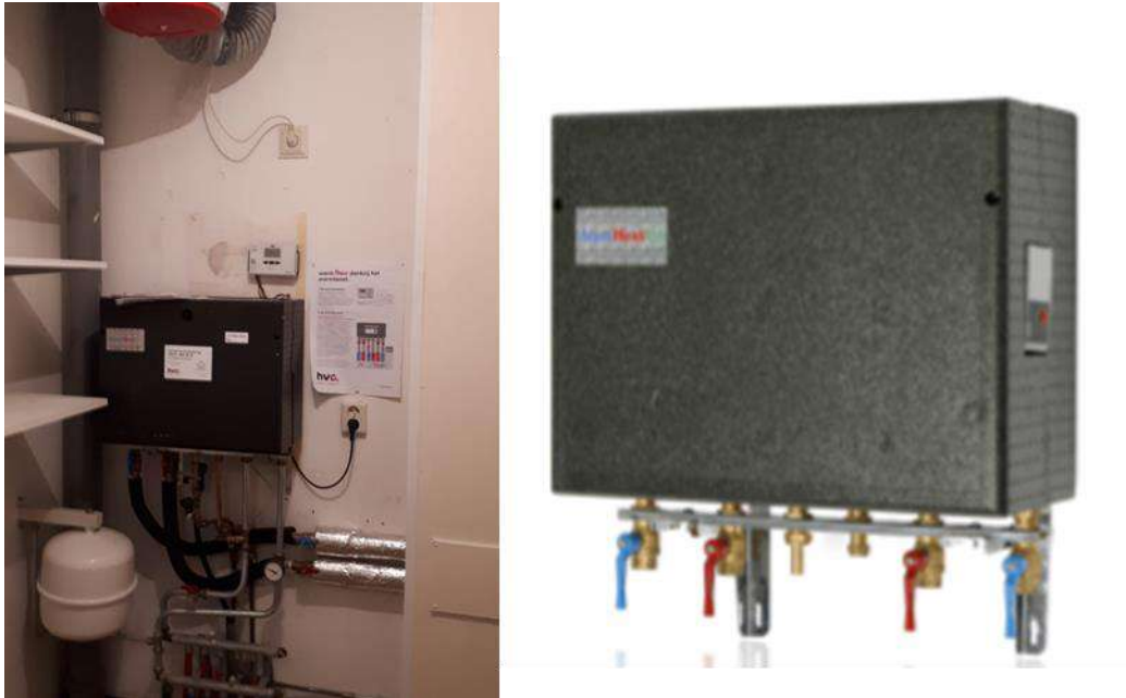
Figure 38: Picture (left) and image (right) of the AquaHeat Arctic-HEX-120 system
