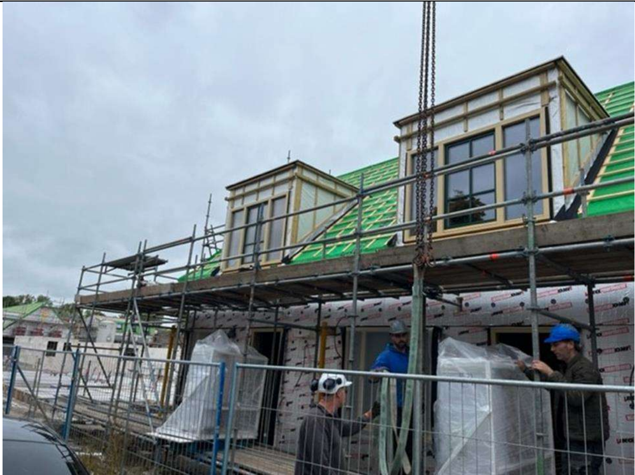
Figure 26: Construction site of houses in Bloemwijk
