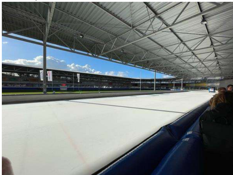
Figure 15: De Meent Ice Rink. On top of the ceiling, 1080 PV panels are installed
