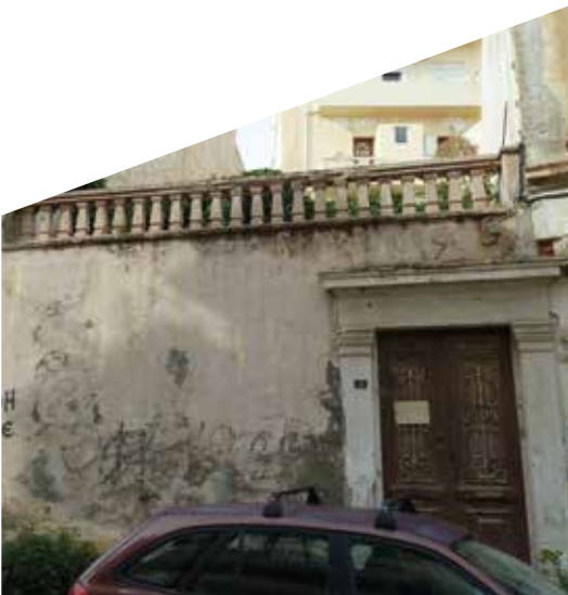
Agia Triada historic district, Heraklion, Greece [TASO Desarrollos SL (photo: Miguel Rivas)]
