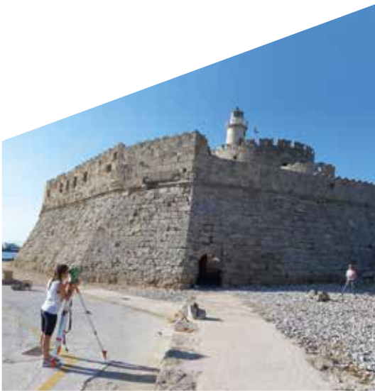
Pilot Site of Rhodes, Fort of St. Nicholas, Greece [Sevasti Tapinaki]
